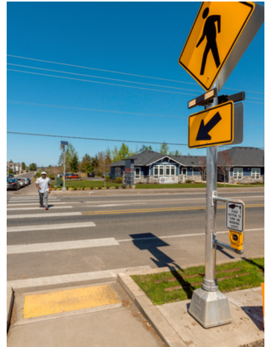
Example of a completed Rectangular Rapid Flashing Beacon (RRFB) crossing, creating a safer and more visible pedestrian crossing.
